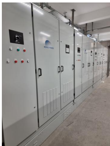
Figure 4 Merus® M2000 STATCOM modules.
